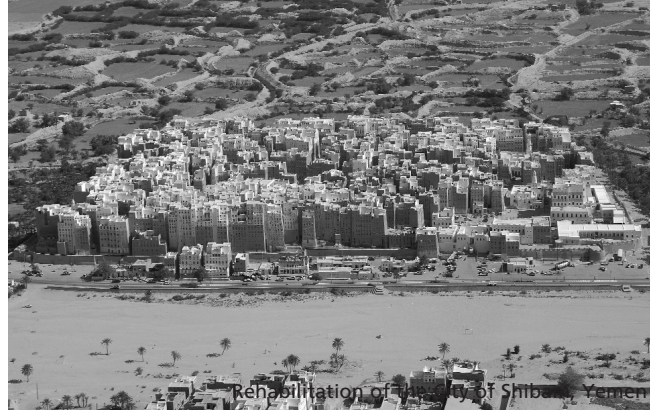
Rehabilitation of the City of Shibam, Yemen
