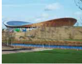
2012 Olympic Velodrome, Hopkins Architects
