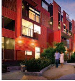
Formosa 1140; West Hollywood, Calif. Lorcan O'Herlihy Architects
