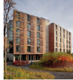
The Housing Tower; Stockbridge, Mass. The Rose + Guggenheimer Studio
