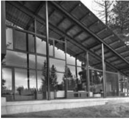
Lake Tahoe Residence
